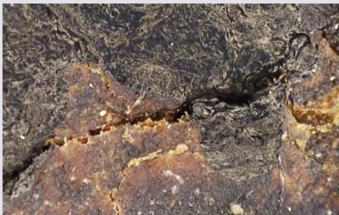
MOTB.SCR.003173 Viscous ink across and into a crack
